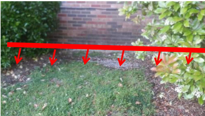
Reconfigure topography near foundation
